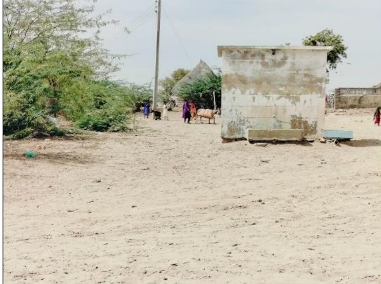
Condition of houses and roads in villages (Field Visit)
